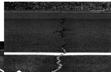
Transverse -Shrinkage of HMA (seasonal changes) -Reflective
