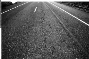
Transverse -Shrinkage of HMA (seasonal changes) -Reflective
