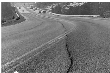
Longitudinal (Joint) -Poor joint construction or location -Reflective
