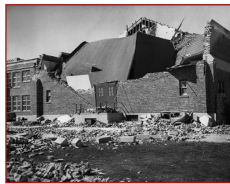
Damage to a School in Long Beach following the March 10, 1933 earthquake 3
