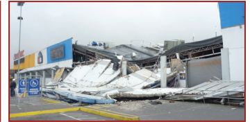
Wall and roof collapse of a Tilt-up concrete buildings
