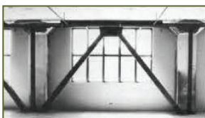
Added Steel Bracing
