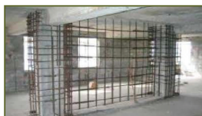
Added New Concrete Walls
