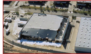
Wall and roof collapse of a Tilt-up concrete buildings
