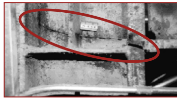
Column flange fracture from the Northridge Earthquake 2 . Roughly 100 SMF buildings had verified structural damage. 3
