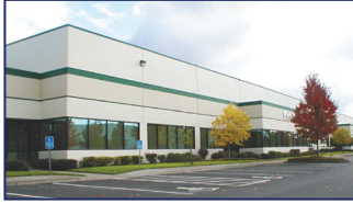
Typical RWFD building (concrete tilt-up)
