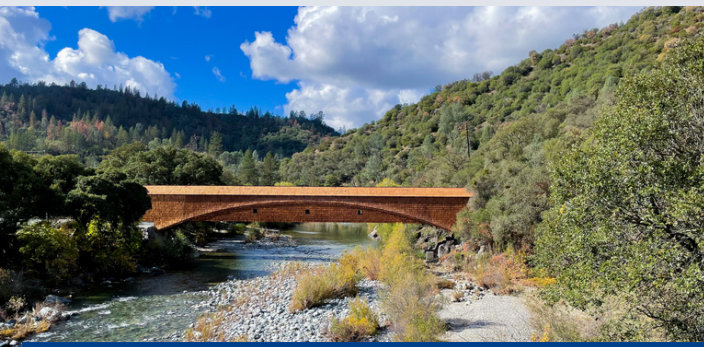
Bridgeport Covered Bridge Buehler Engineering Excellence - Historic Preservation
