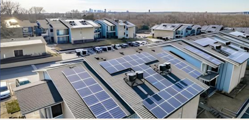
Transforming multi-family homes with cost-saving solar PPAs
