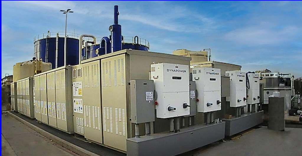
RedFlow 2MWh ZnBr Installation Dec. 2021, California
