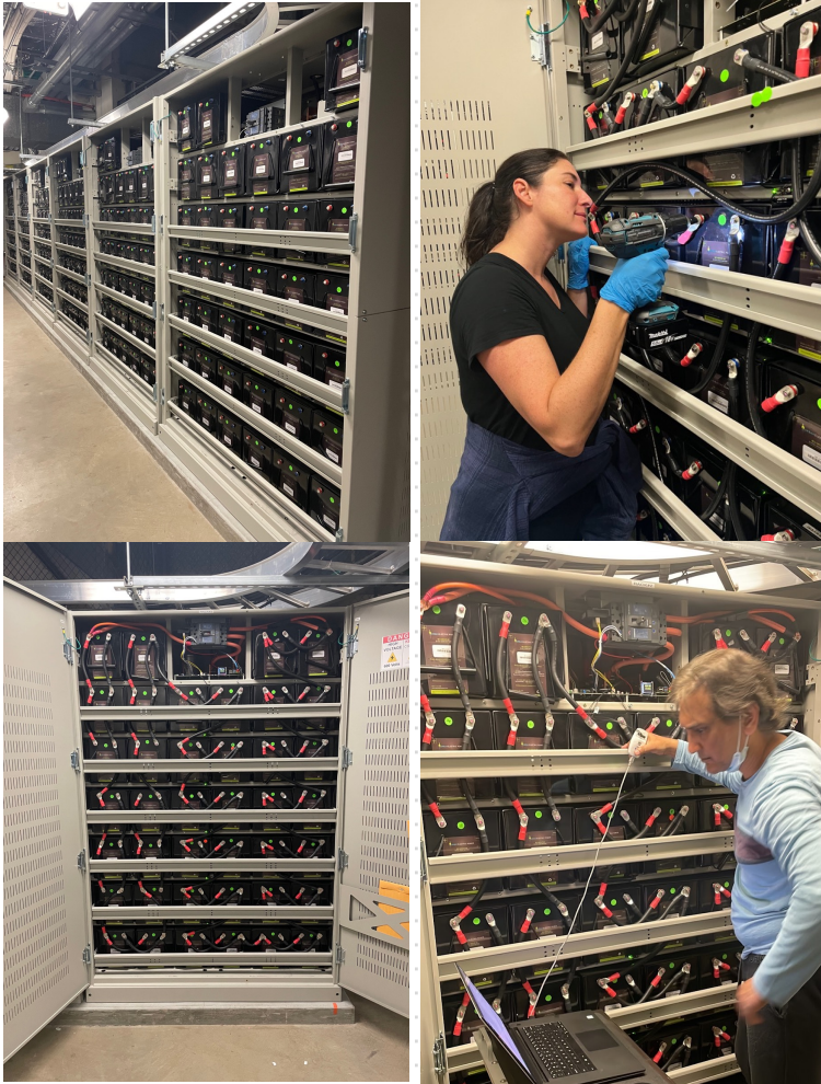
Layout for the San Diego Supercomputer Center 1MW/2MWh Backup System
