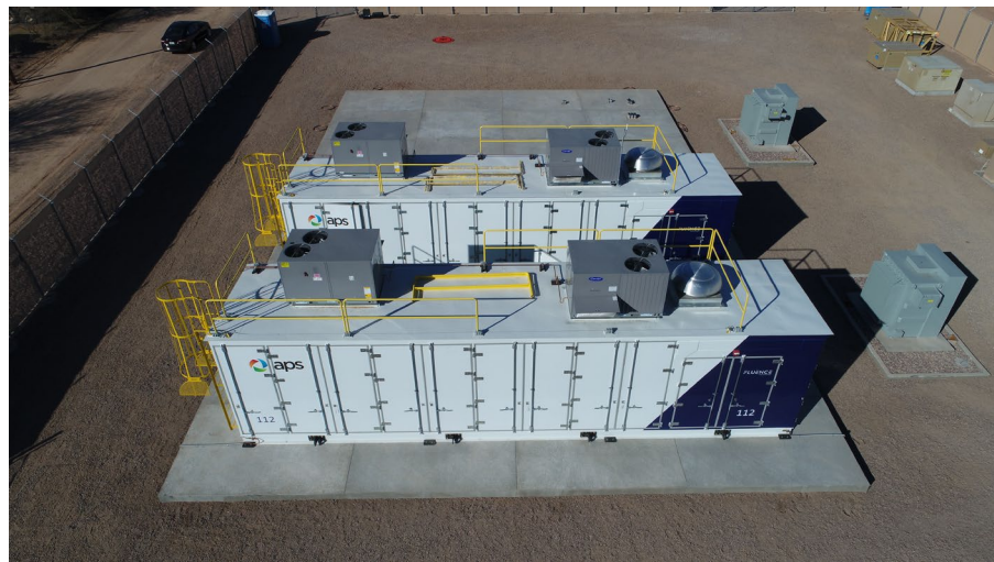
Two BESS Containers (1MW/4MWh each)
