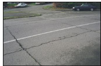
**Possible Causes:** Movement of the concrete slab beneath the asphalt surface because of thermal and moisture changes, or shrinkage cracking in the subgrade and reflection up through the surface layers, or too thin of flexible pavement surface. Generally not load initiated, however loading can hasten deterioration.
