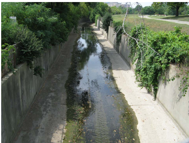
Figure 9. Sections of the Clinton River flow through concrete banks. Water levels can be very high or low because the river receives a lot of urban runoff.
