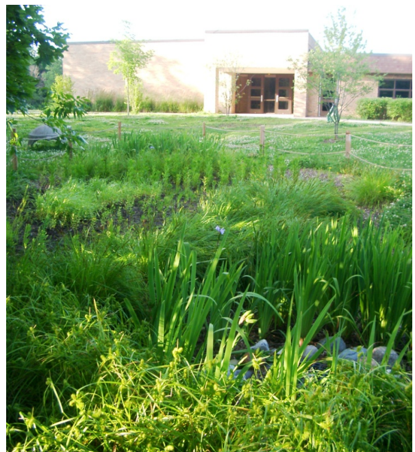
Figure 12. A rain garden that captures water from the roof of an elementary school in Ann Arbor, Mich.
