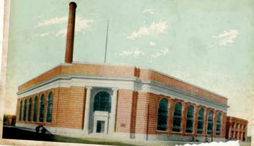
231. Filtration Plant, Grand Rapids, Mich.
