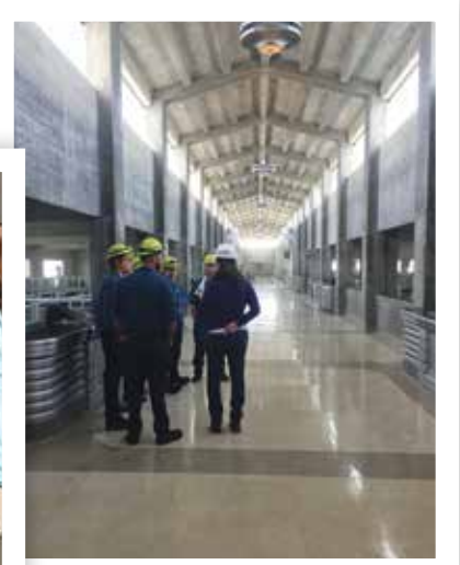
Plant employee, Cindy Irving, explaining the sand filtration process
