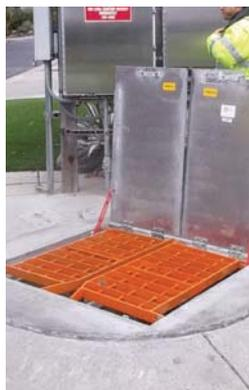
EJ aluminum access hatches are designed to provide easy and secure access to below ground infrastructure, and feature stainless steel hardware.
