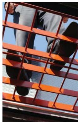
SAFE HATCH® safety grates cover the opening and provide fall through protection in conformance with OSHA standard 1910.23.
