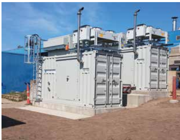
Twin KB 100 Biogas CHP Modules Pictured above
