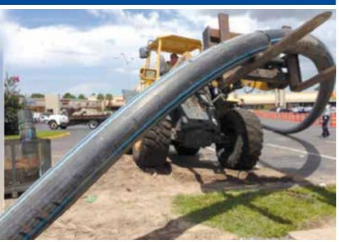
With superior seismic resistance, HDPE piping systems are also the material of choice for trenchless installations due to fused joints, flexibility, high ductility, qualified contractors, and many other features and benefits.
