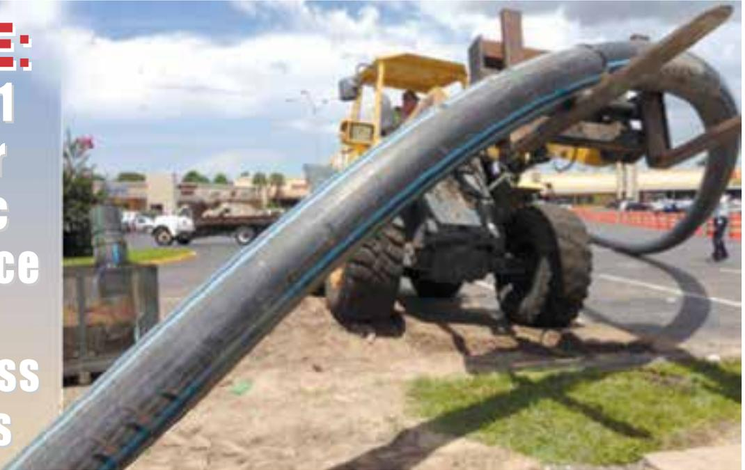
With superior seismic resistance, HDPE piping systems are also the material of choice for trenchless installations due to fused joints, flexibility, high ductility, qualified contractors, and many other features and benefits.
