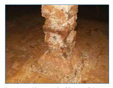
Deteriorated Reservoir Roof Support Column
