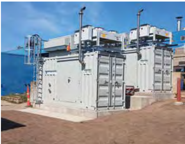
Twin KB 100 Biogas CHP Modules Pictured above
