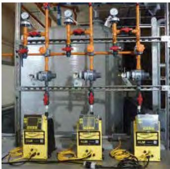
The EXCEL® XR metering pump is a mechanically actuated diaphragm pump driven by advanced variable speed technology to provide the most accurate and reliable performance in the industry.
