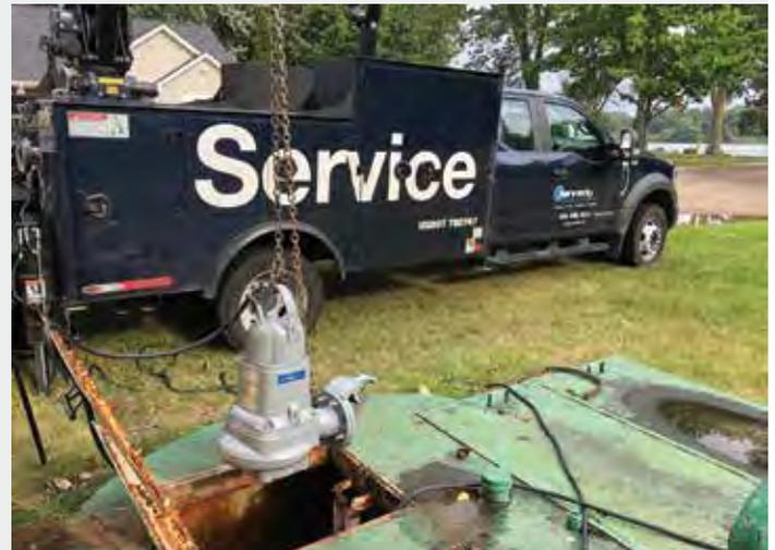
Flygt Concertor's discharge design allowed it to be installed with the existing manufacturer's guide rail bracket.
