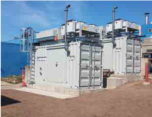
Twin KB 100 Biogas CHP Modules Pictured above
