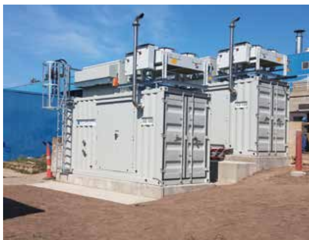
Twin KB 100 Biogas CHP Modules Pictured above
