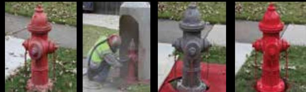
BEFORE PREPARATION    DURING PREPARATION    PREPPED FOR PAINTING    COMPLETION OF PAINT
