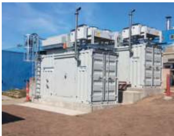
Twin KB 100 Biogas CHP Modules Pictured above
