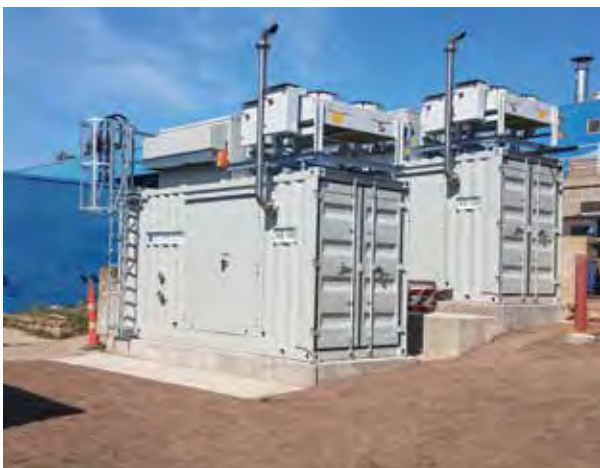
Twin KB 100 Biogas CHP Modules Pictured above
