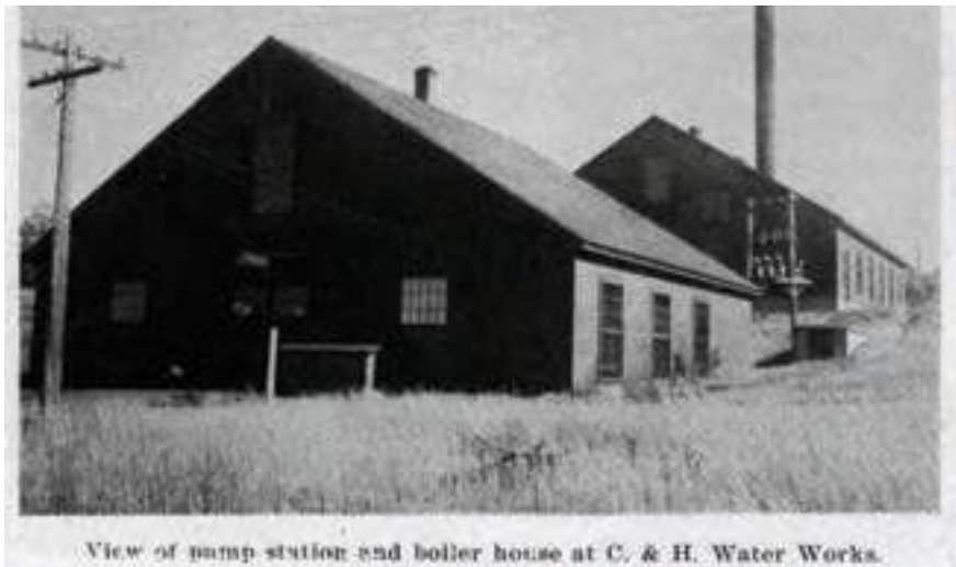
In this photo from 1945, the photographer takes a photo of the exterior view of the pump station and boiler house at C&H Waterworks.
