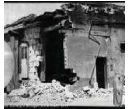
In this photo taken June 17, 1976, titled "Death of a Landmark," demolition work was started late last week on the old Baraga Water and Electric Building, which had been a part of the village since 1912. Replaced by a modern water plant a few years back, the building was deemed to have outlived its usefulness and was condemned by the village council a few months ago. The image is of the rundown building about to be destroyed.
