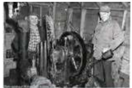
The Redridge Community's water supply came from a pump at the Baltic Mill. Here Henry Hiltunen and his son Earl attend the pump. Water came from an artesian well in the hillside nearby. Though the mill closed in 1922, Copper Range supplied water free to all residents till 1962. A fire pump in the boiler house supplied high-pressure water from the steel dam to fight fires but through the same pipeline. Date of Photo: 1960-1970.
