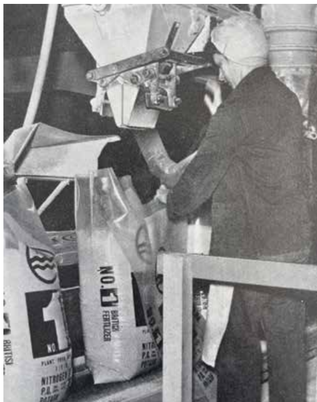
Conventional, manual filling via push-on spouts from a Reifenhäuser system at the customer ICI, England
