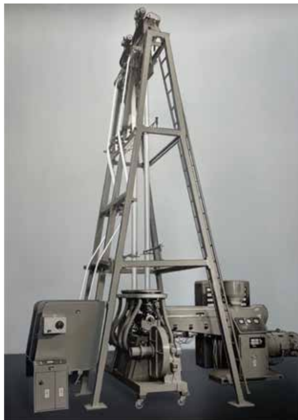
Reifenhäuser’s first blown film lines with vertical extruder
