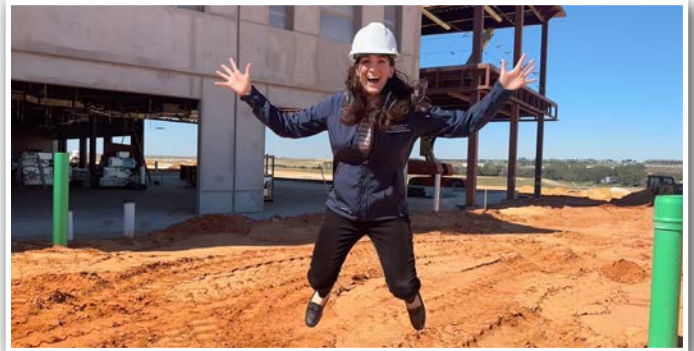
Above: FOMA DS-3 Trustee Samantha Cotler, DO, MBA tours the OCOM construction site
