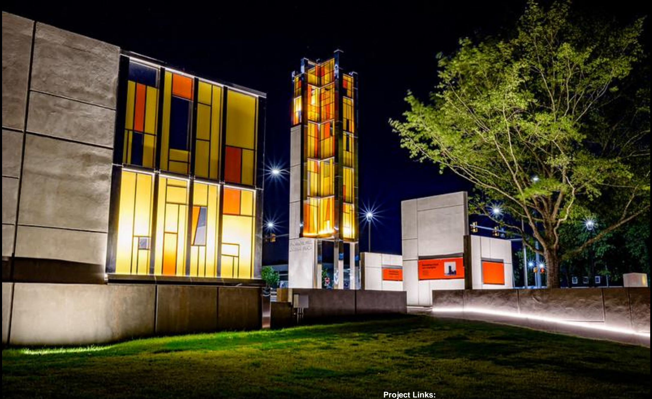
An iconic tower creates a dynamic beacon at the corner of First & Greene Street which symbolizes the former stained glass church bell tower.
