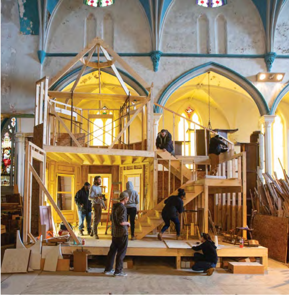
Tradition and Innovation. The SACRA Quarter House Project (above) demonstrates building techniques common to Victorian-era architecture within the city of Buffalo while the SACRA Building Arts Library (left) features contemporary design approaches, including the use of structural insulated panels and reclaimed materials.
