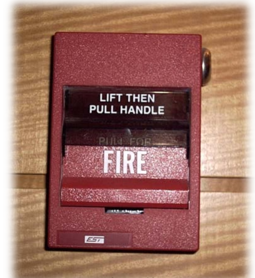
Manual Pull Station
