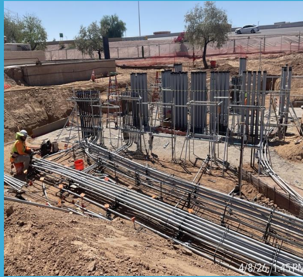
Lift Station 40 Refurbishment – Electrical Building Conduit - Construction Services
