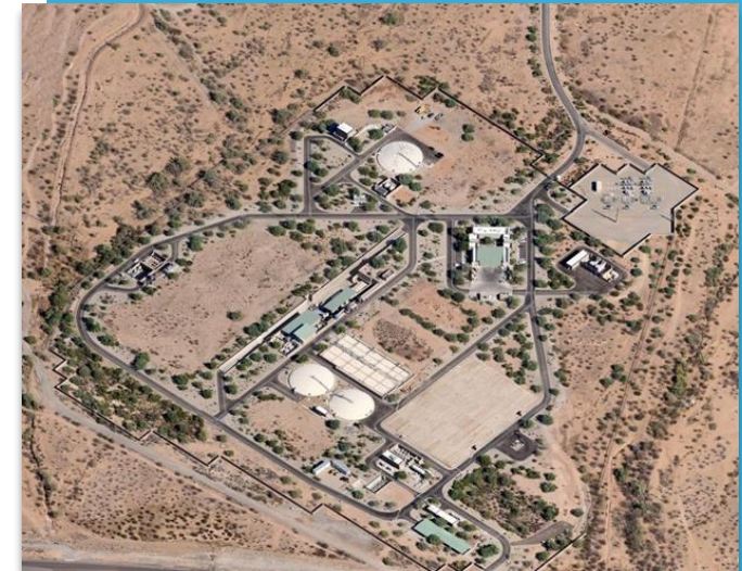
Cave Creek WRP (Built in 2000, currently being rehabilitated)
