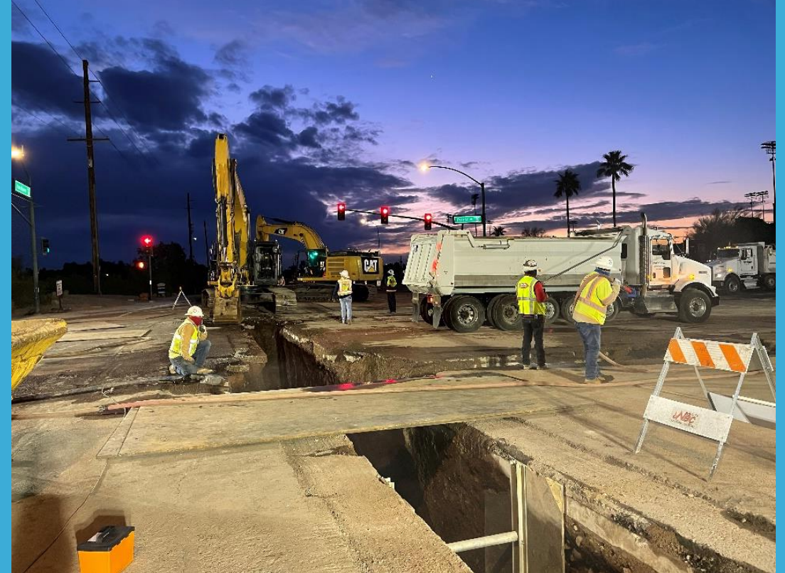
Trenching for a New Sewer Line
