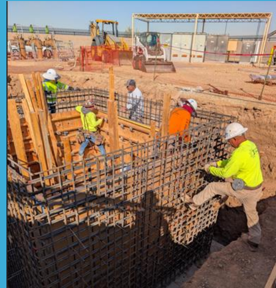
Lift Station 73 – New Biofilter Installation – Construction Services
