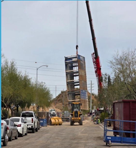
51 st Avenue Gravity Sewer – Construction Services
