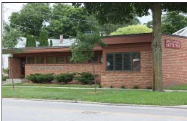
Building where Dr. Gimer's practice is located in Iowa Falls, IA.
